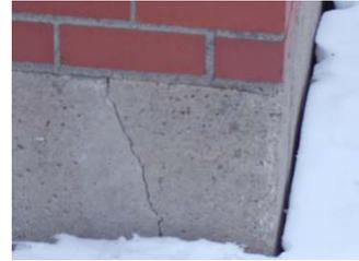
**Recommendations:** The areas of cracking and control joints should be cleaned of debris and the cracks and control joints should then be sealed with appropriate concrete crack filler and sealed.
